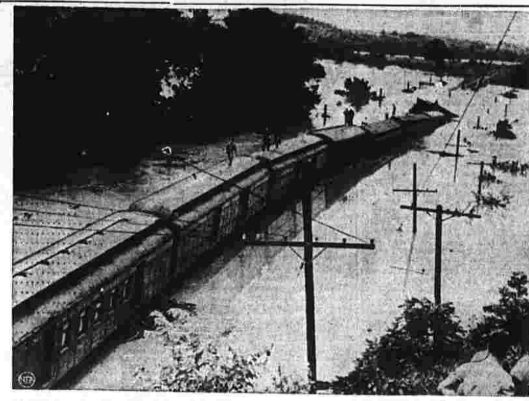
In that partially submerged Missouri Pacific passenger train, wrecked when rain-swollen Joachim Creek near Festus, Mo., washed out a section of track, Engineer W. W. Mulloy was believed to have died by drowning. Five cars and the engine were derailed in the accident, the locomotive overturning and the train was marooned for hours until the flood subsided sufficiently for rescue workers to reach the scene.
